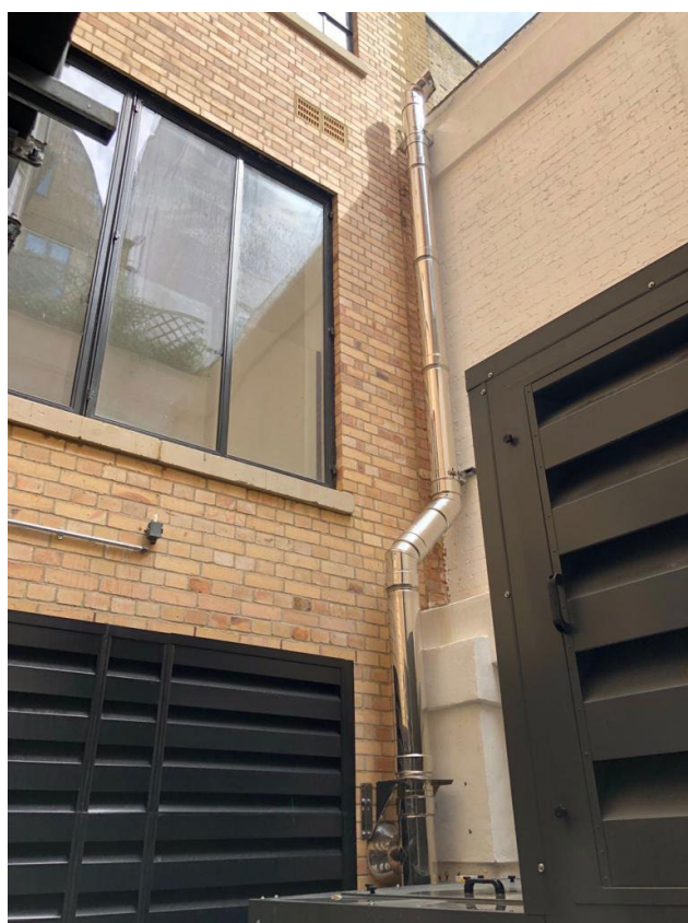
Generator exhaust flue
